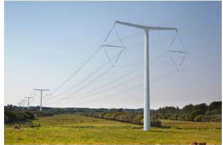
T-pylon / Photo: National Grid
