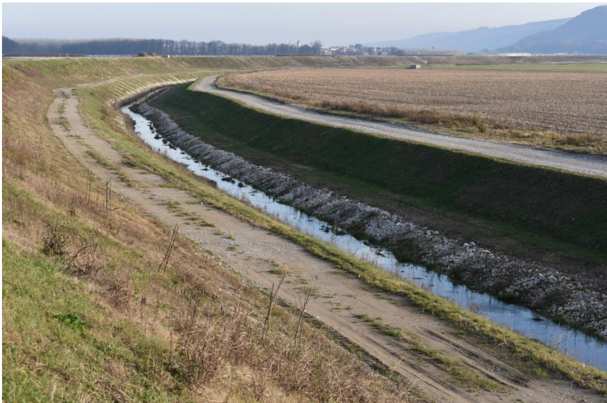
Figure 49: The drainage channel on the right bank has not been constructed sustainably as habitat for rheophilic fish species.
