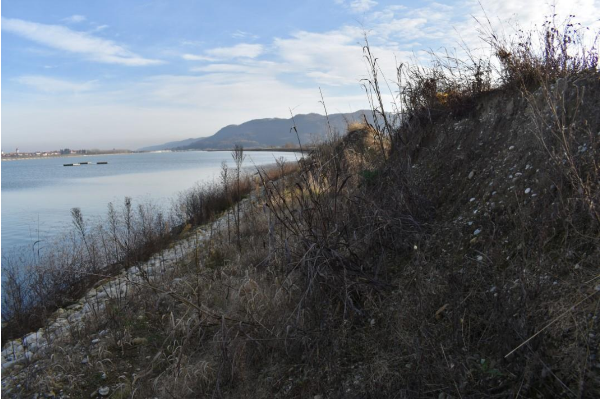
Figure 37: The banks are not maintained and are, in turn, covered by overgrowth.
