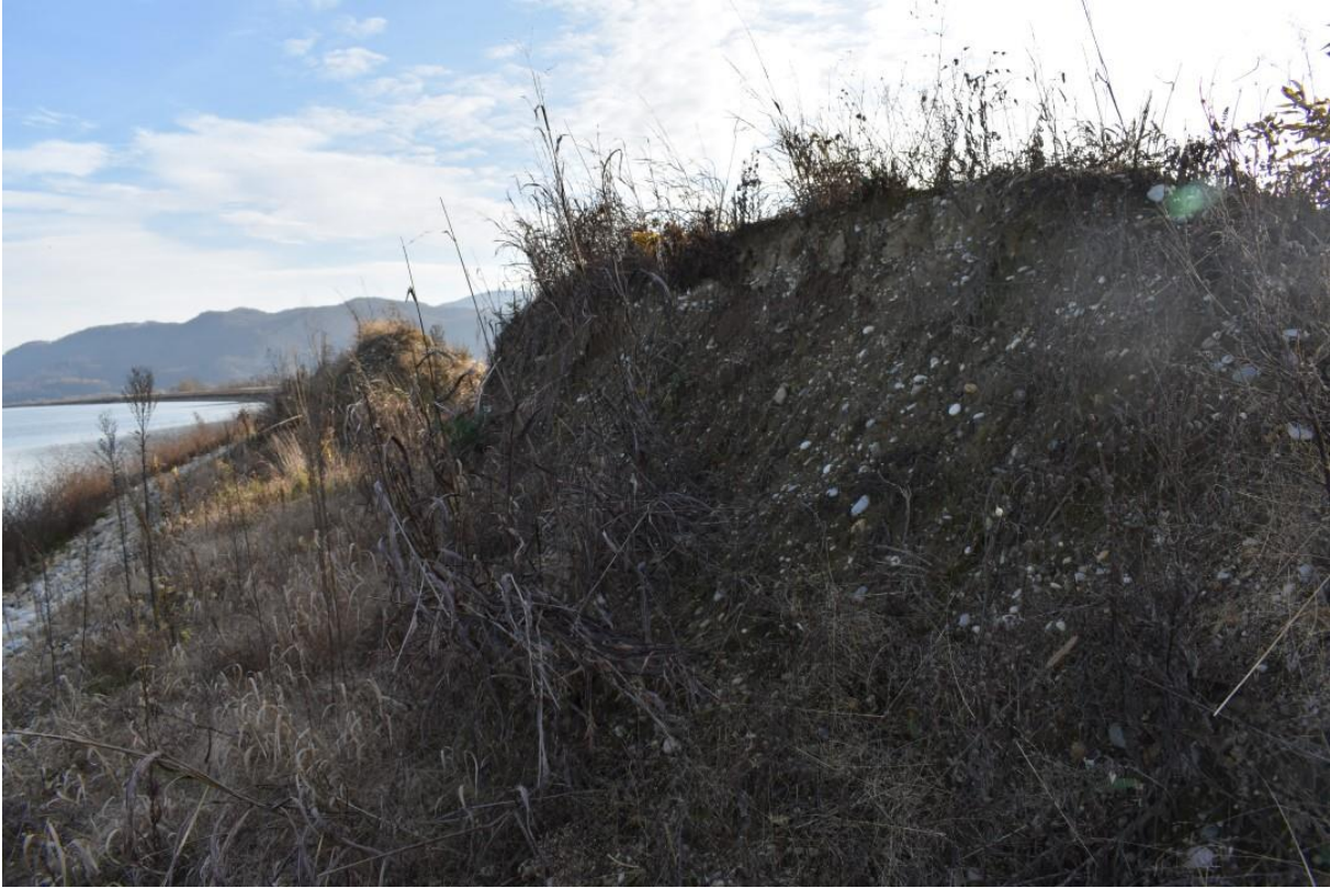
Figure 36: The banks have been built of unsuitable material.
