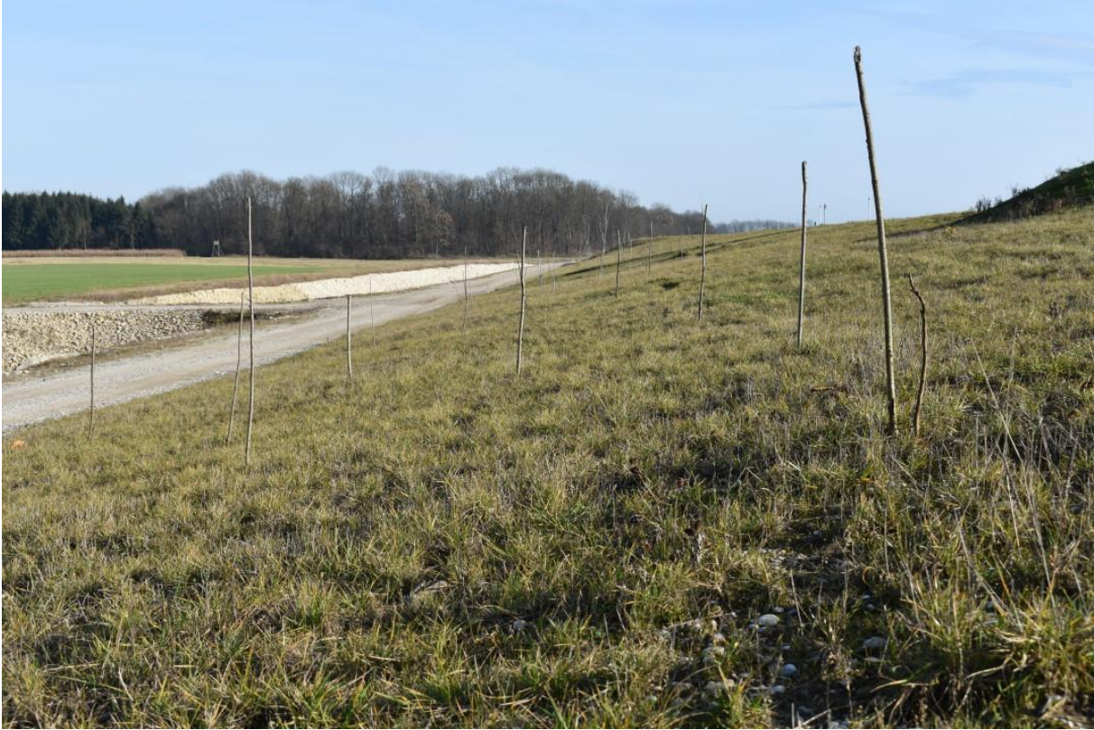
Figure 50: Planting attempt proved to be a complete failure.
