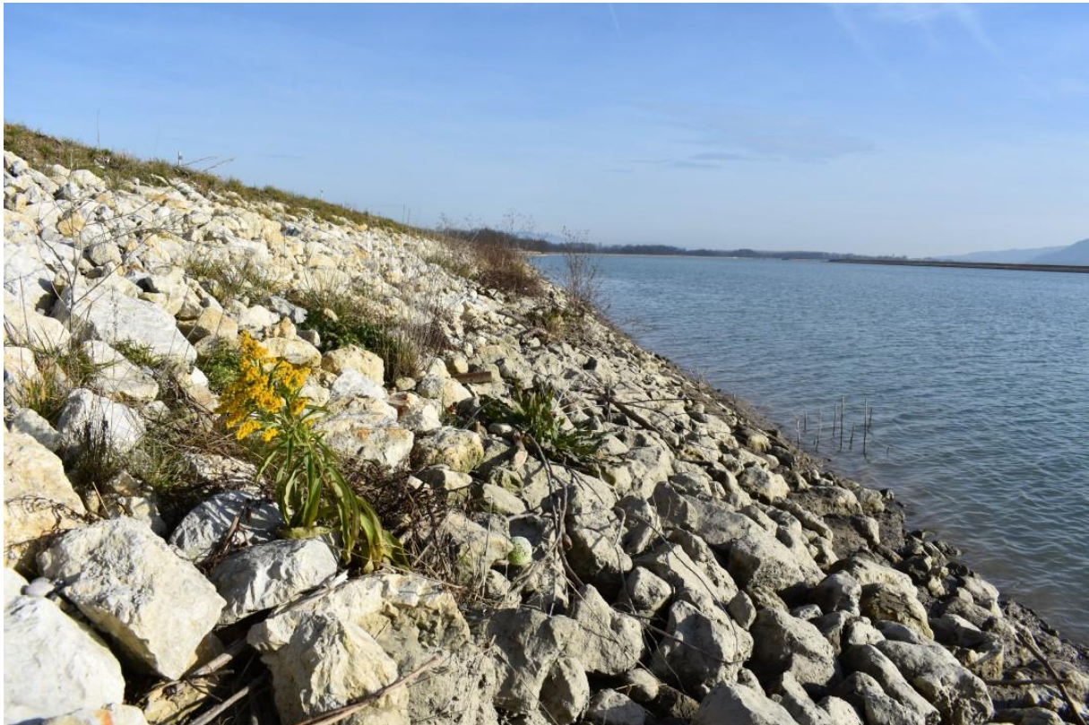
Figure 53: The banks are fortified with composed stones and not planted with vegetation; in places, the invasive Goldenrod ( Solidago sp. ) can already be seen.
