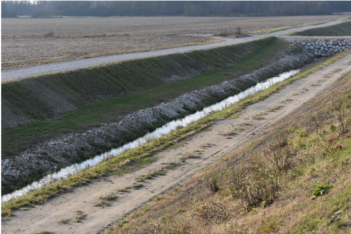
Figure 47: The drainage channel on the right bank has not been constructed sustainably as habitat for rheophilic fish species.
