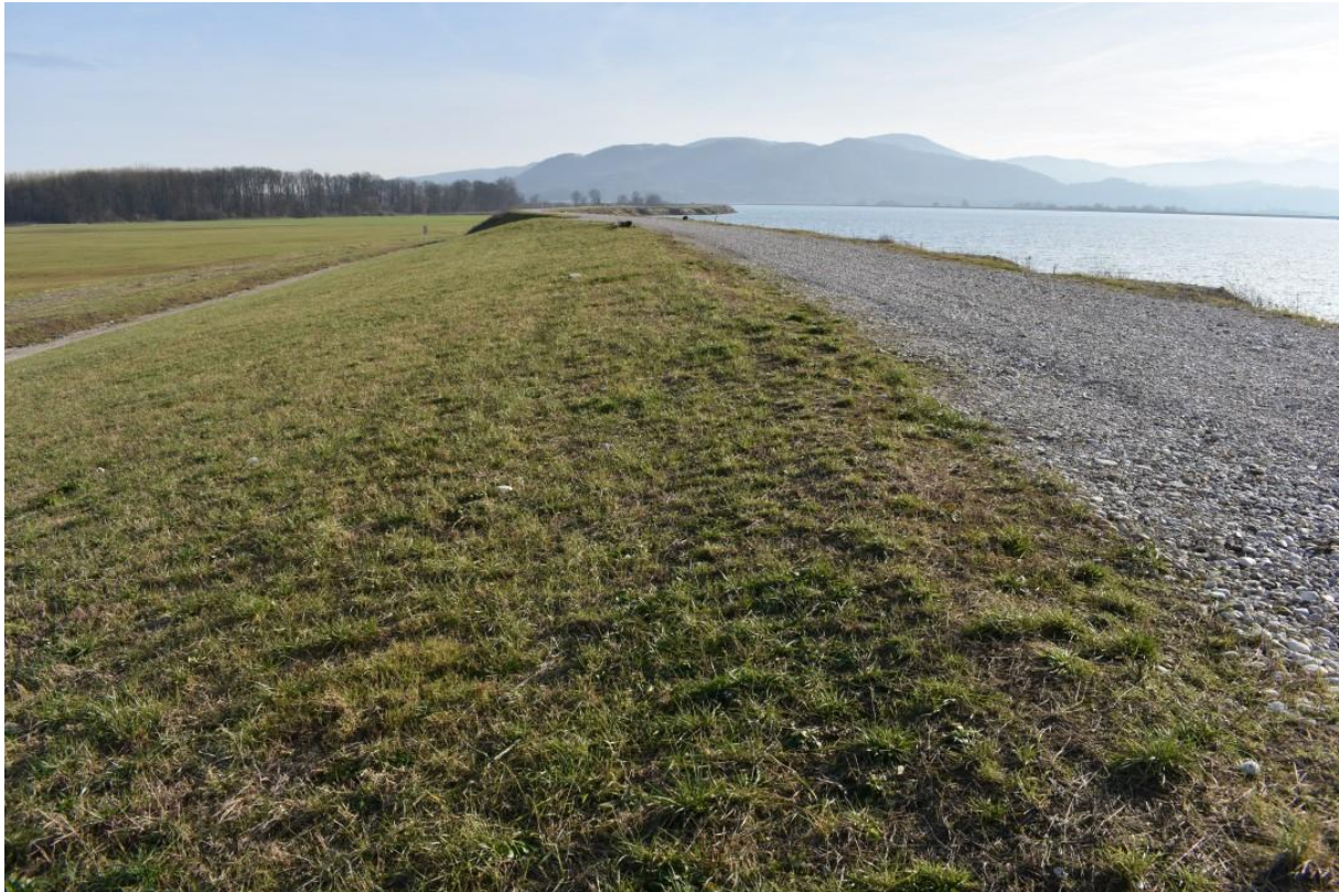
Figure 2: Widening of the flood protection embankment
