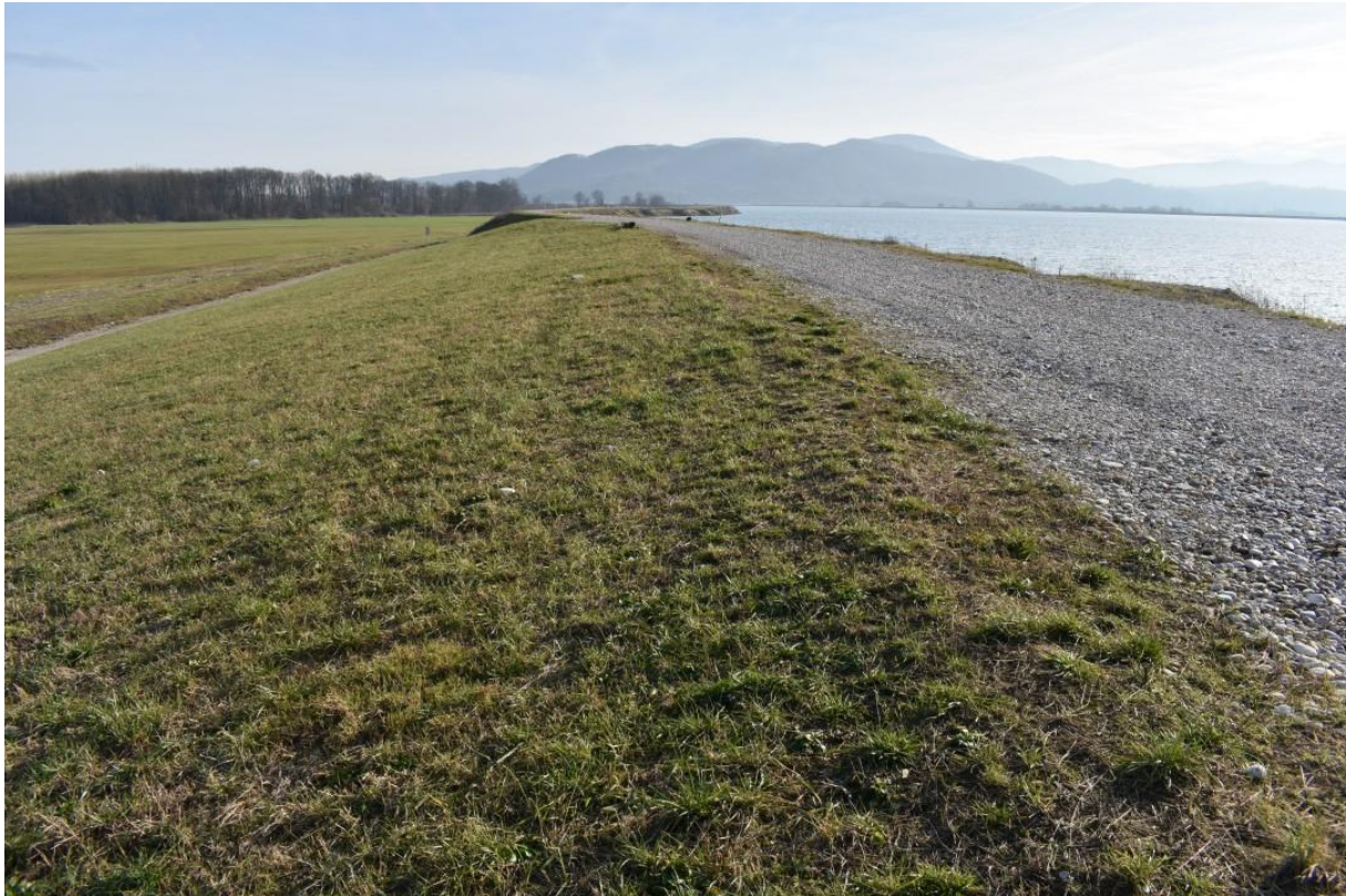
Figure 55: The widened parts of the embankment have not been planted with shrubs and trees.
