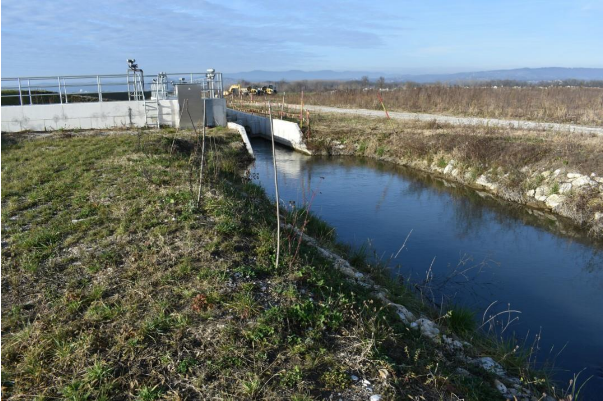
Figure 6: Failed attempt at planting shrubs and trees, with passage for water dependent organisms in the background
