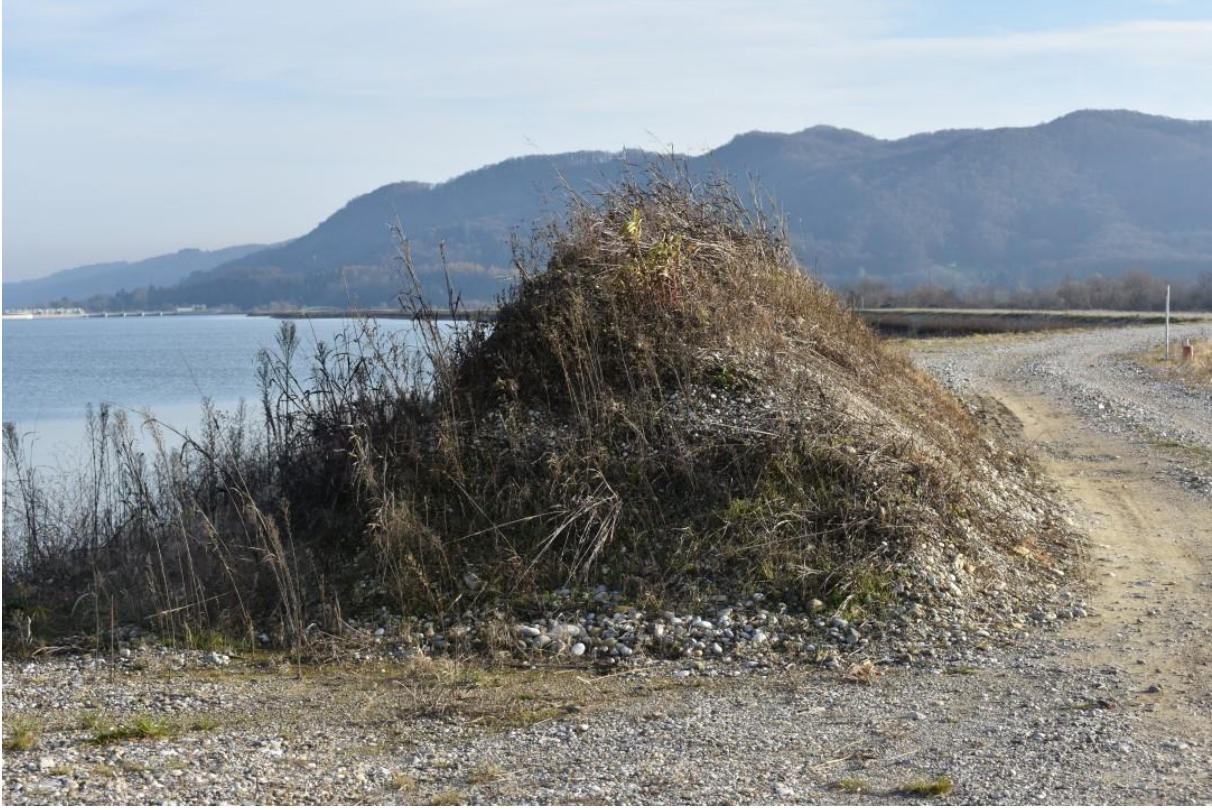
Figure 35: No shrubs have been planted behind the banks.
