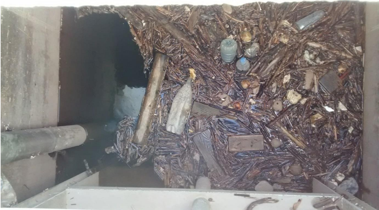
Figure 7: Passage between the fish pass and reservoir, where waste is accumulating
