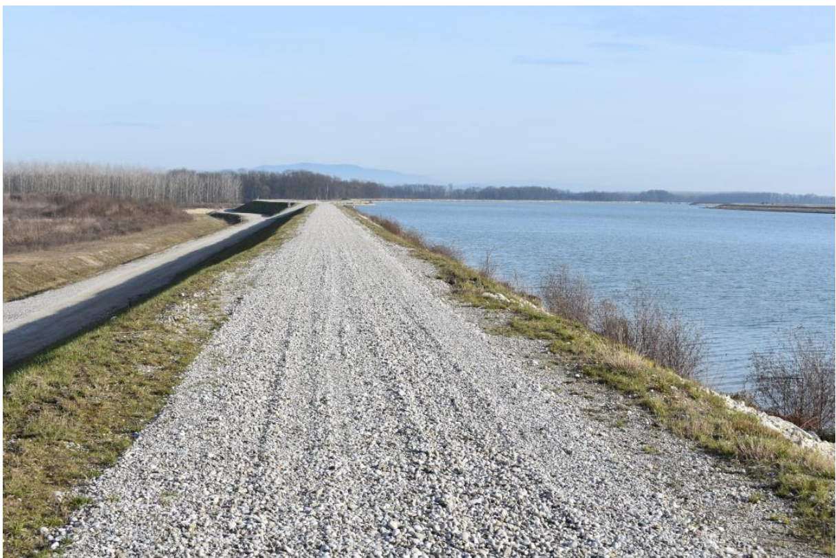
Figure 54: Greening of the upper parts of consolidated banks with autochthonous plants has not been carried out.
