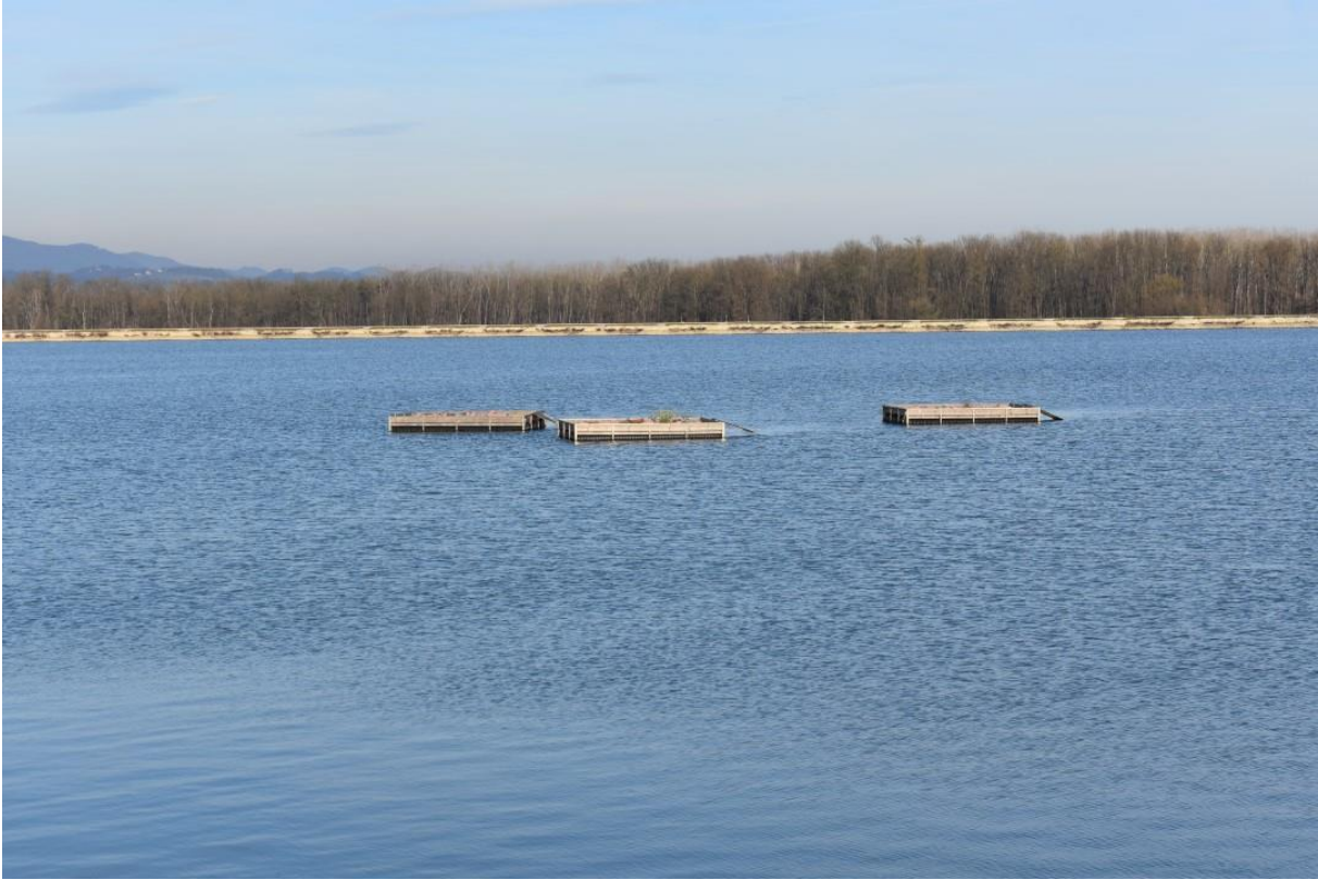
Figure 42: For breeding terns, 3 floating rafts were constructed
